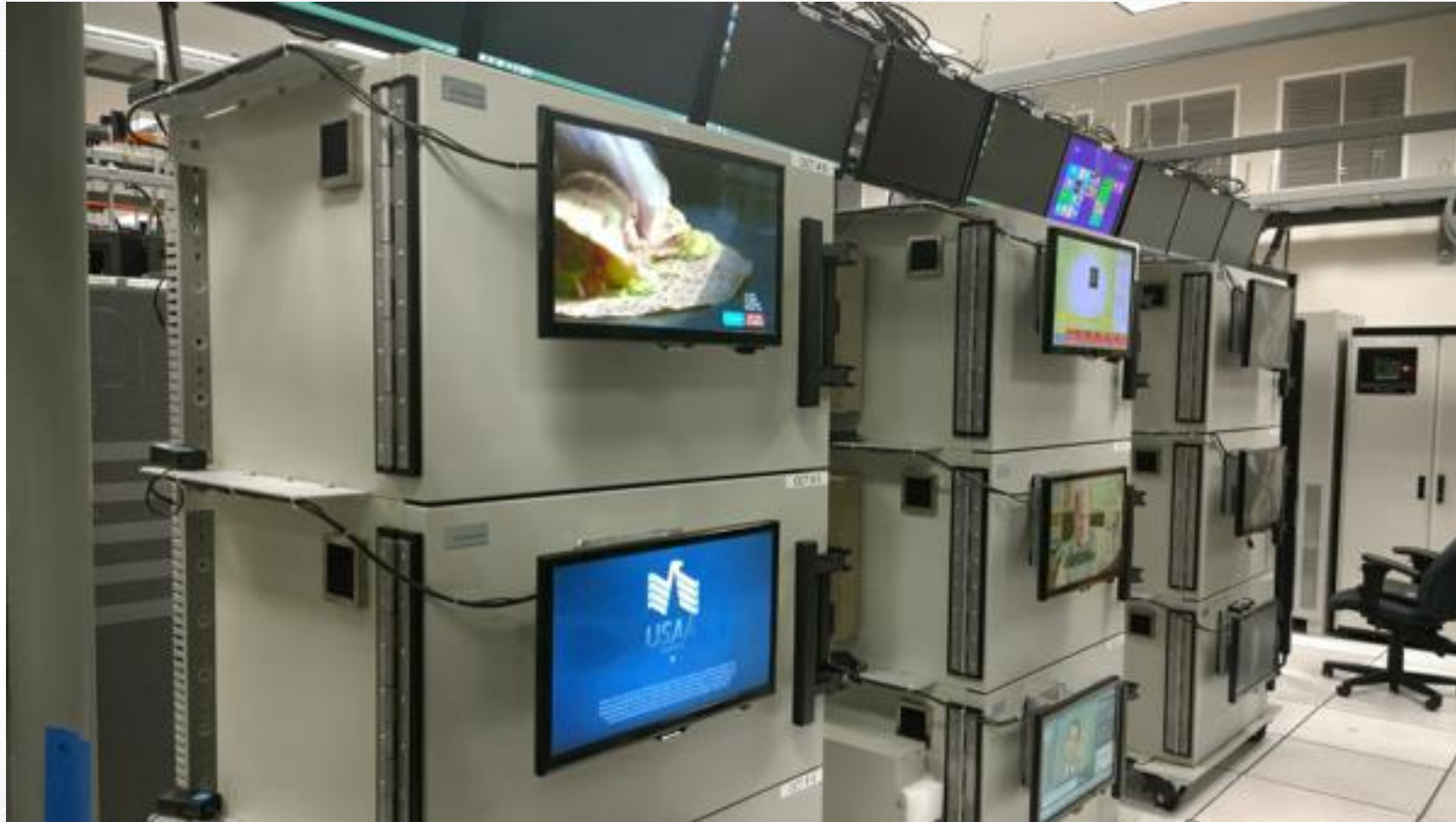
Video, data over Wi-Fi testbed
